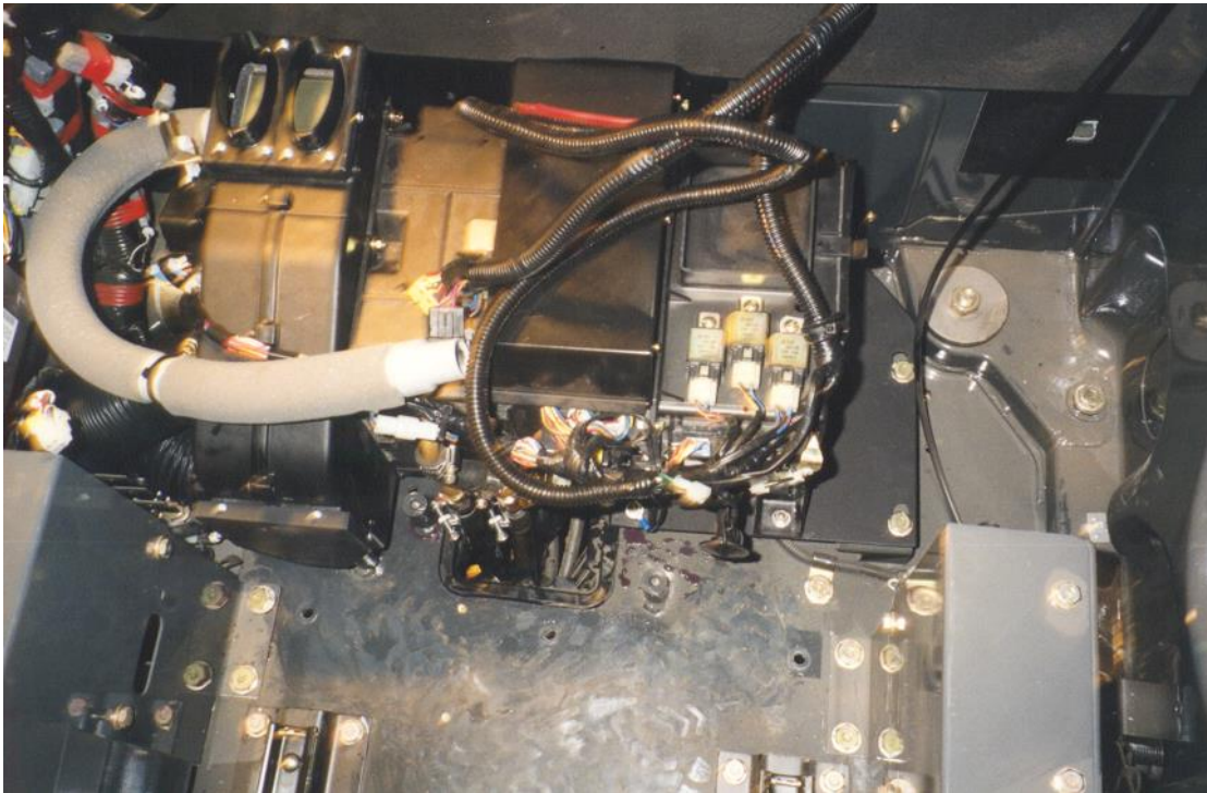
Evaporator assembly mounted in place.
